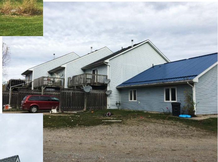
Figure 8. Rear View of Quadplex
