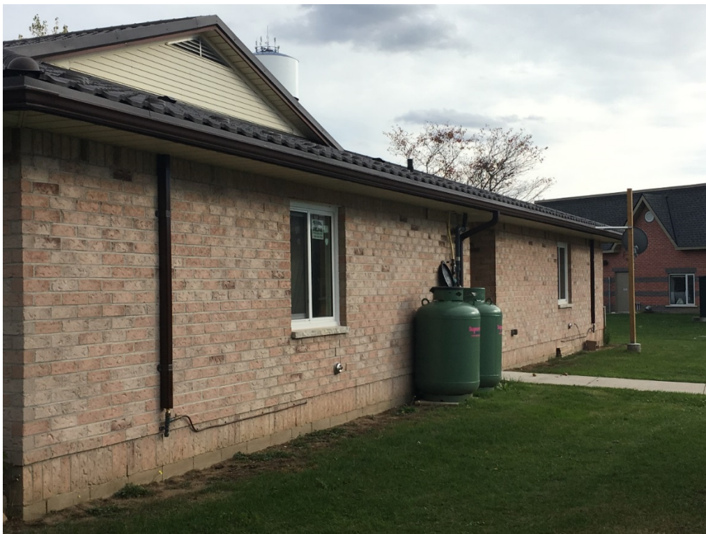
Figure 4. Side View of Senior Citizens Complex with Propane Tanks
