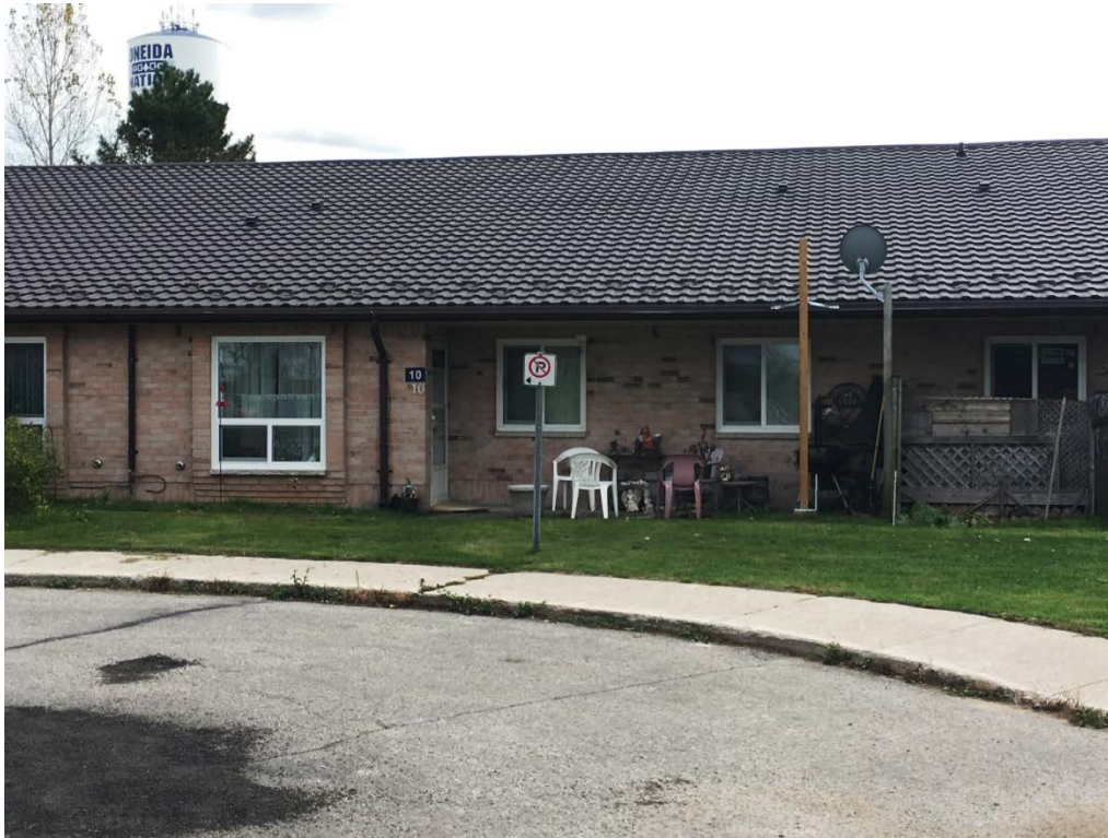
Figure 3. View of Front Individual Units of Senior Citizens Complex
