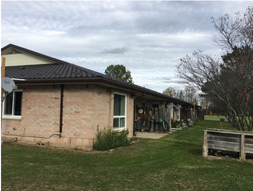
Figure 5. View of the Back Units of the Senior Citizens Complex
