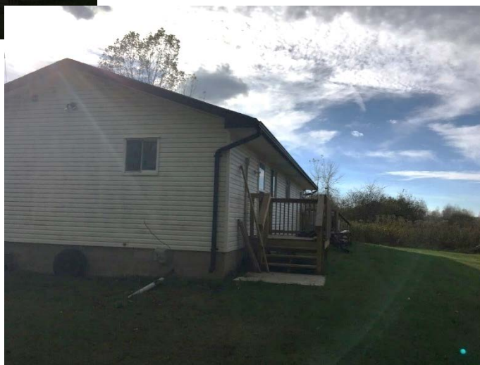
Figure 11. Duplex: Side and Back View
