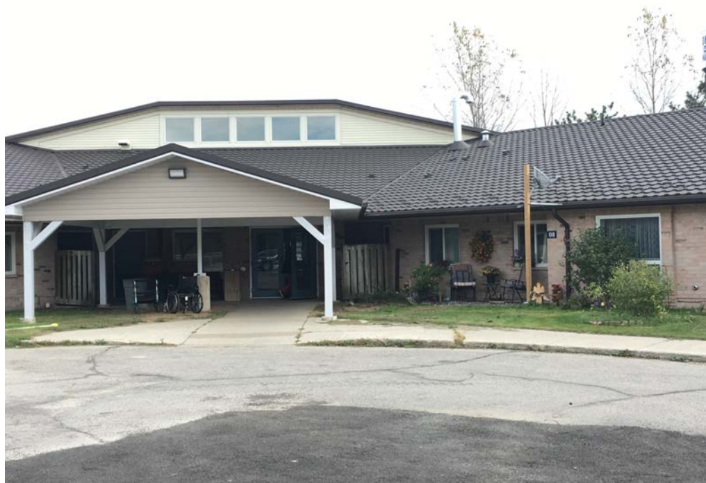
Figure 2. Front View of Entrance Senior Citizens Complex
