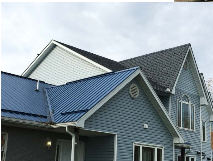
Figure 9. Quadplex Roof: Metal and Asphalt Shingles
