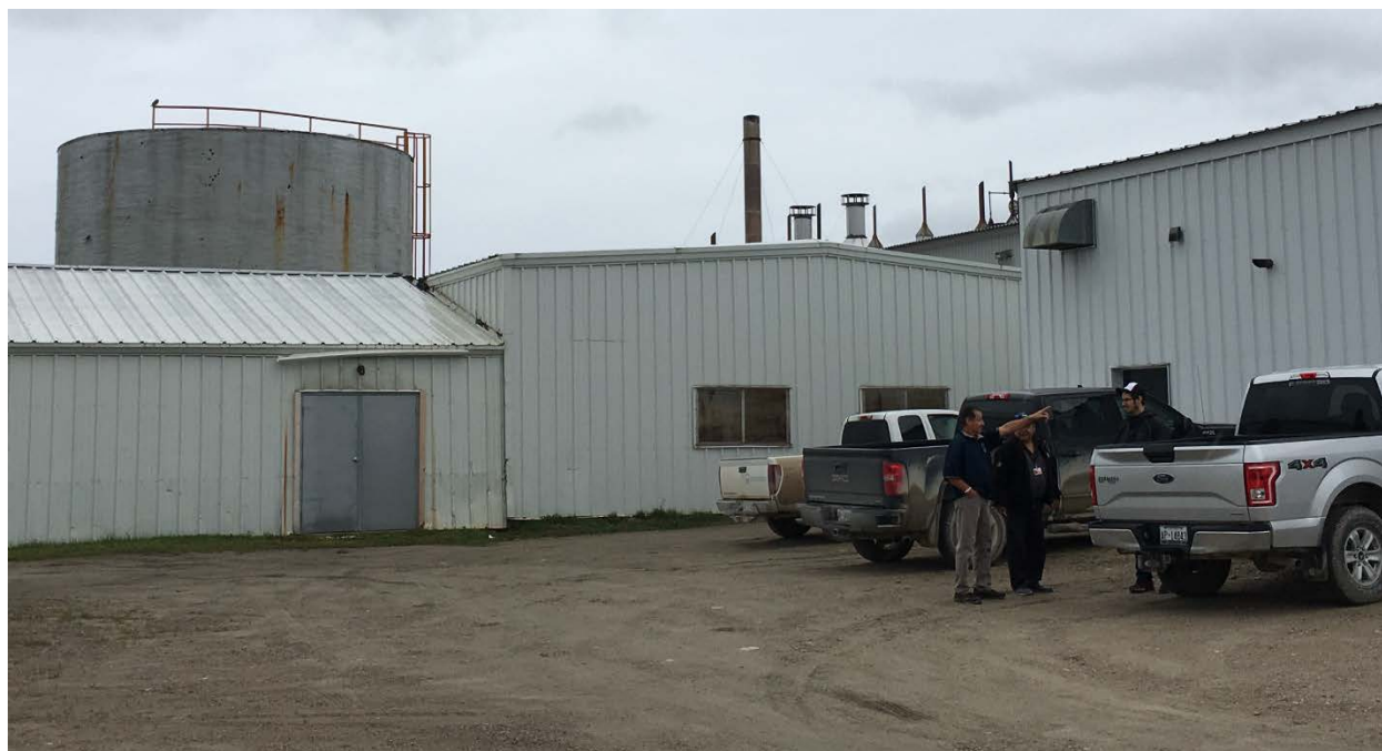
Figure 5: Photo of Water Treatment Plant Building and Reservoir taken during the September 26, 2017 Site Visit as part of Workshop 1
