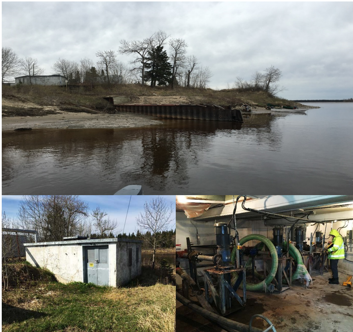
Figure 7: Raw Water Intake and Low Lift Pump Building
