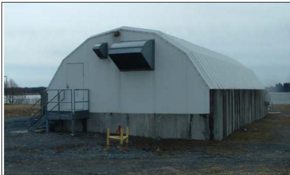
Figure 12: Exterior View of Block 97 RBC
