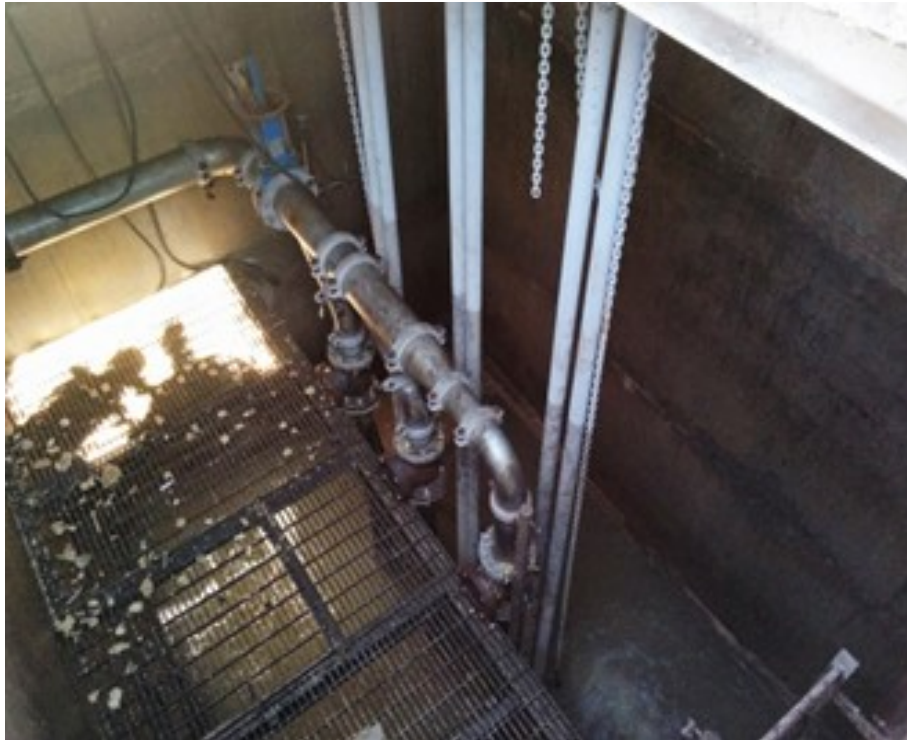
Figure 20: Interior of the Cherry Street Pump Station
