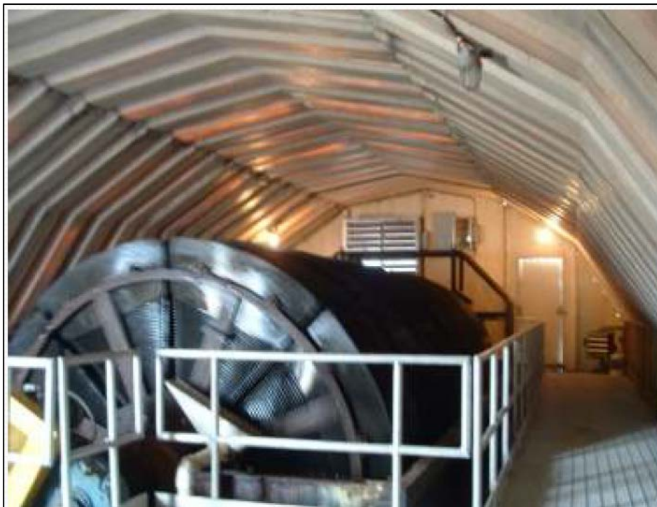
Figure 13: Interior View of Block 97 RBC
