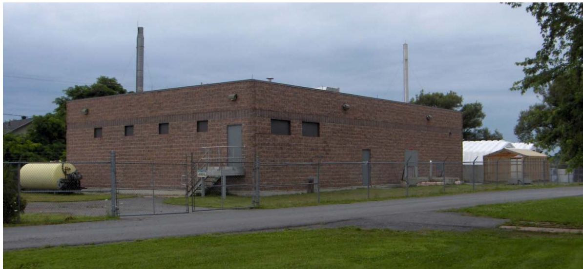
Figure 21: Exterior View of the St. Regis Wastewater Treatment Plant
