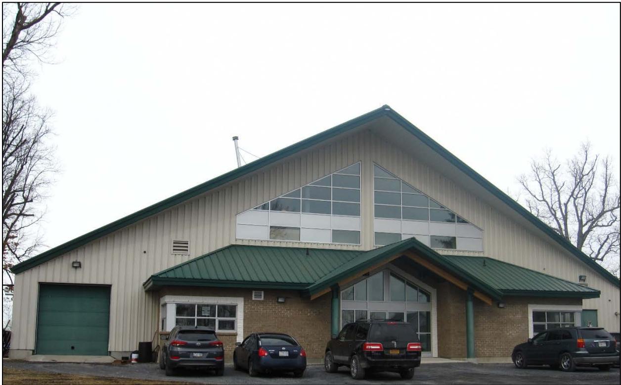
Figure 7: Cornwall Island Water Treatment Plant Building
