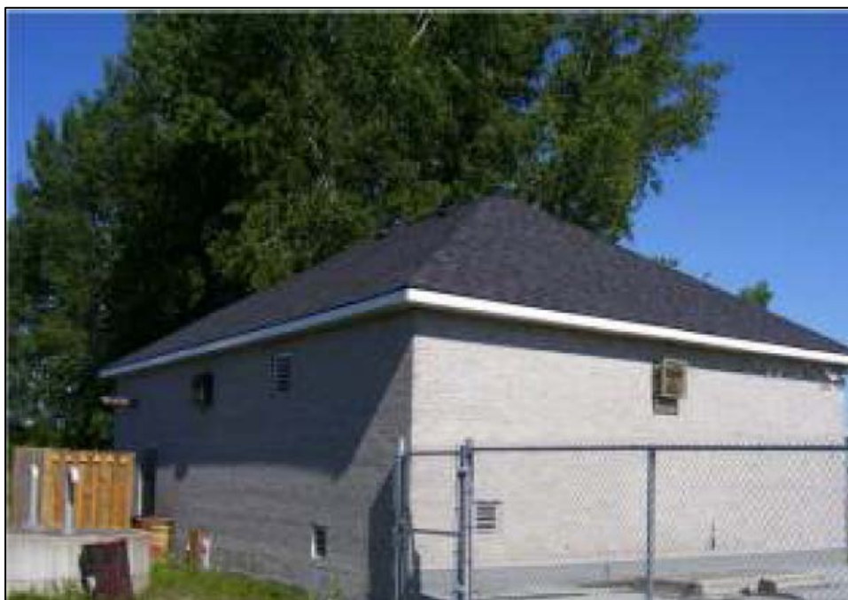
Figure 15: Building of the High Lift Station at Block 97
