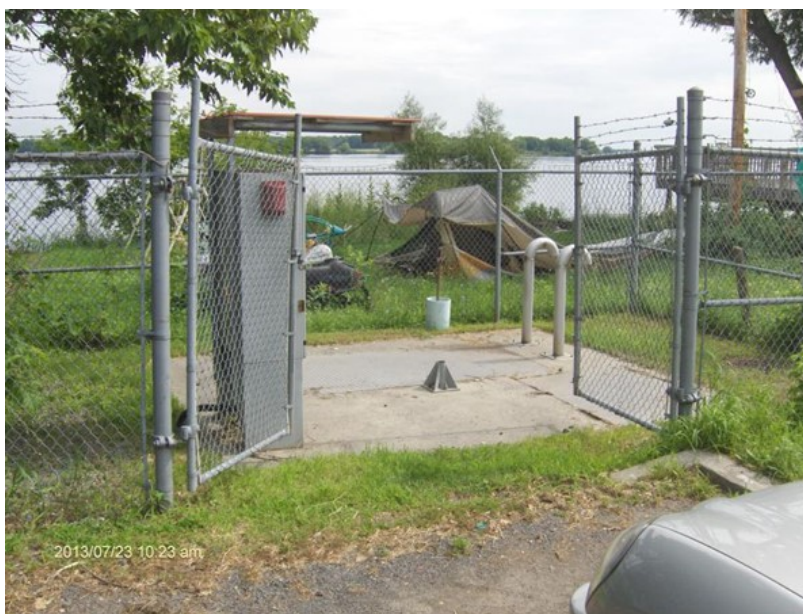
Figure 19: Exterior of the Cherry Street Pump Station
