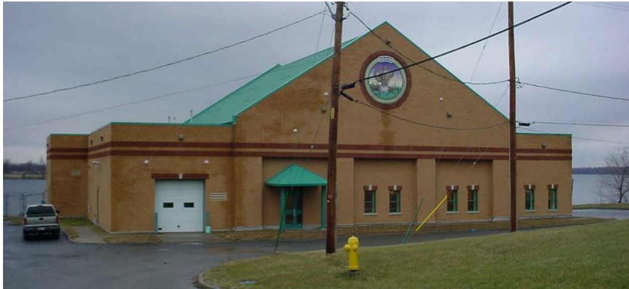
Figure 17: Exterior View of the St. Regis Water Treatment Plant
