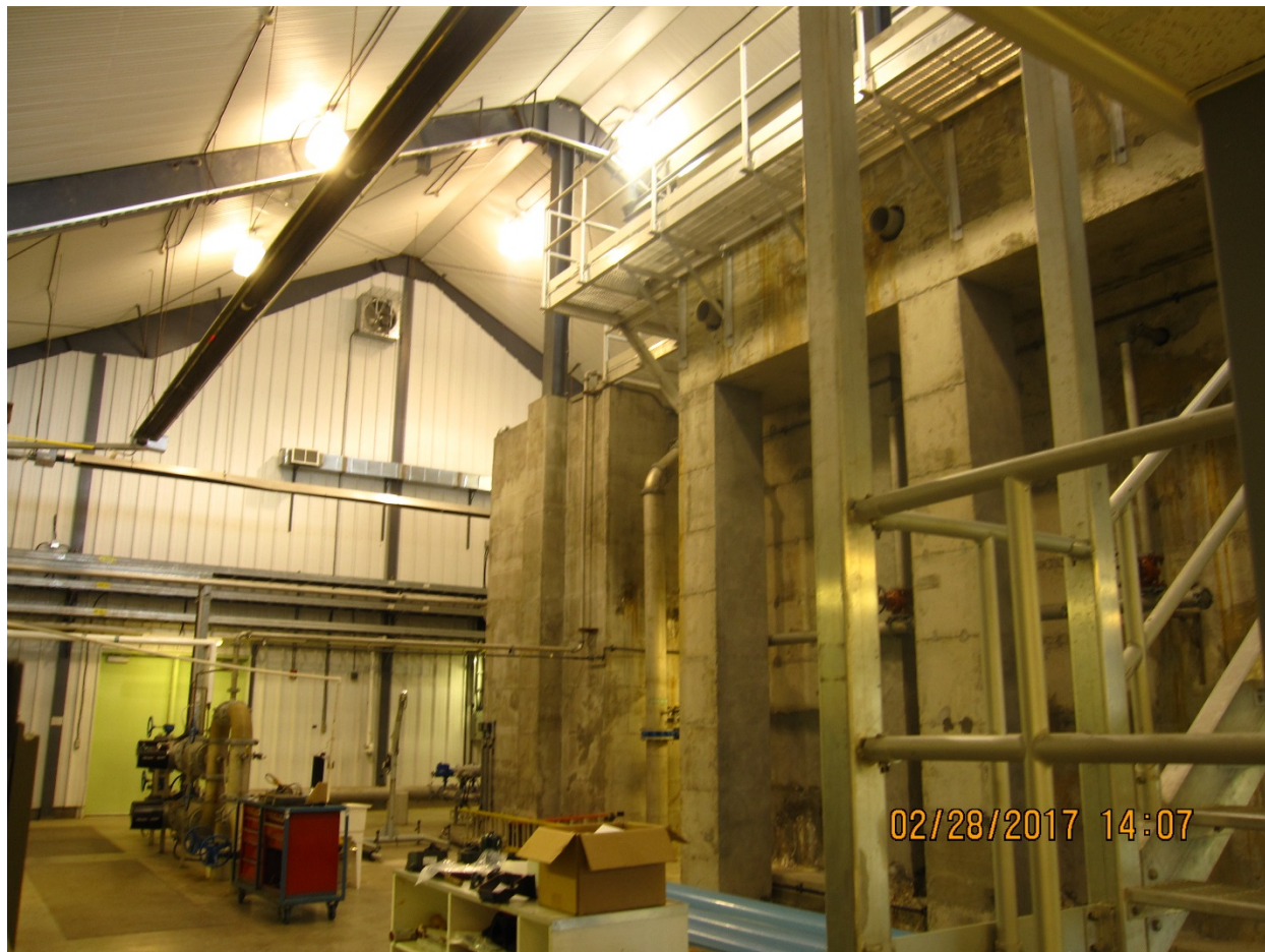
Figure 9: Inside View of the Cornwall Island WTP
