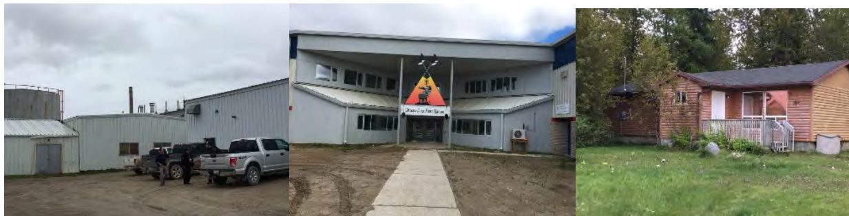
Photos: Water Treatment Plant, Government Offices, Residential House, Site Photos
